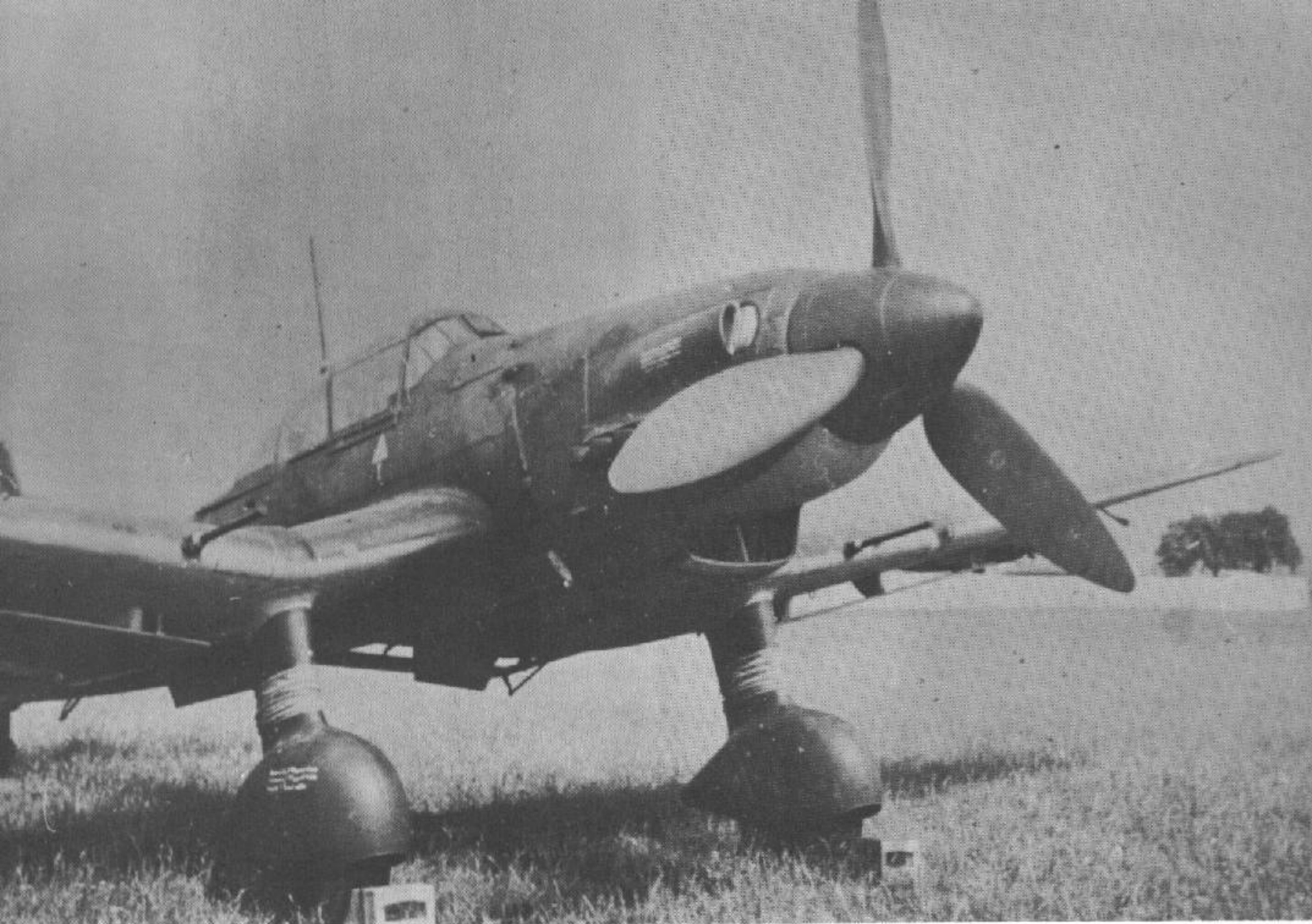
Junkers Ju 87 D-7 supplied to the Slovakian Air Force for service on the Eastern Front. The Ju 87 D-7 version had two wing-mounted 20 m m. MG 151 cannon.
