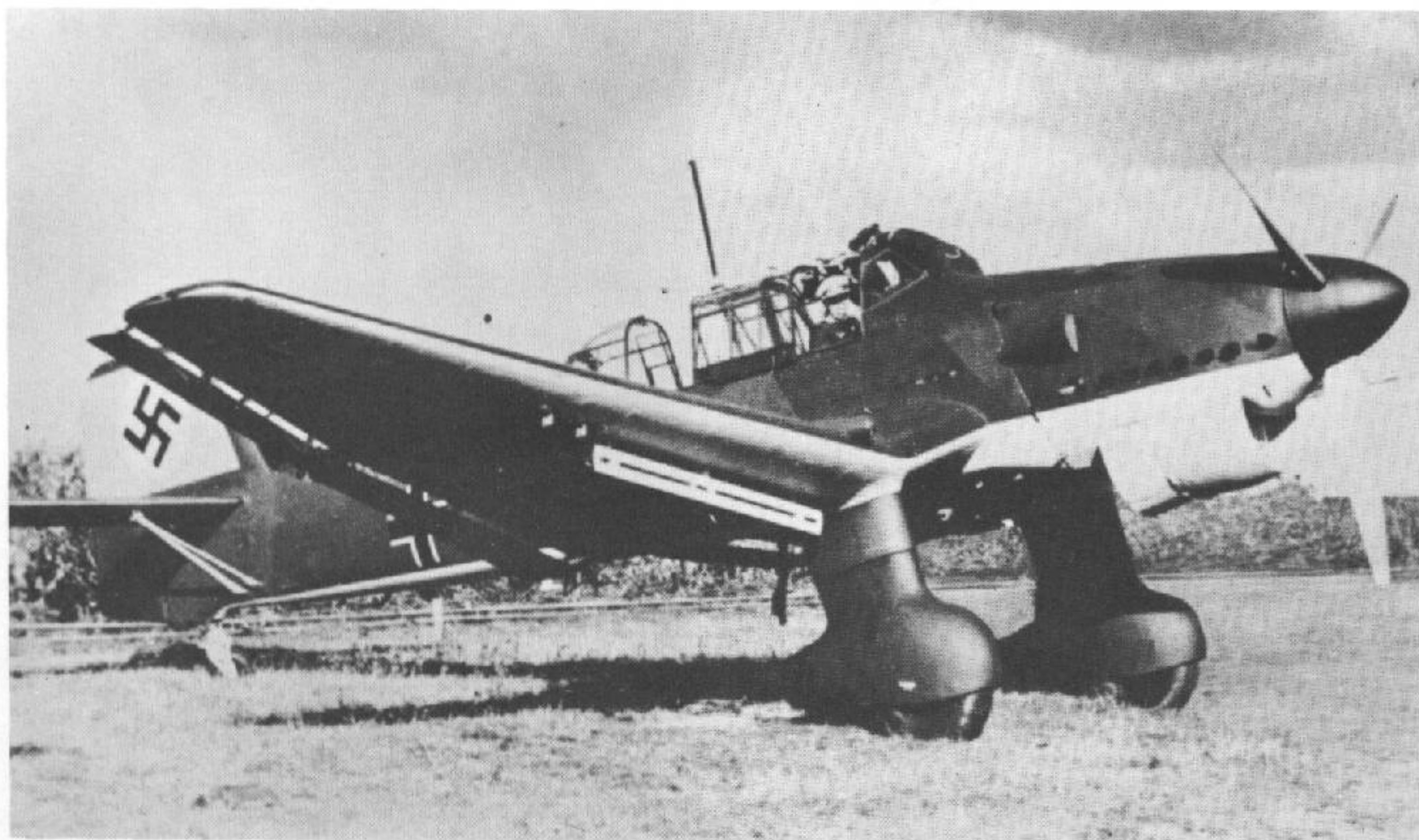
Early Ju 87B-1 production model prepared for acceptance flight. Note extended Dive Brake.
