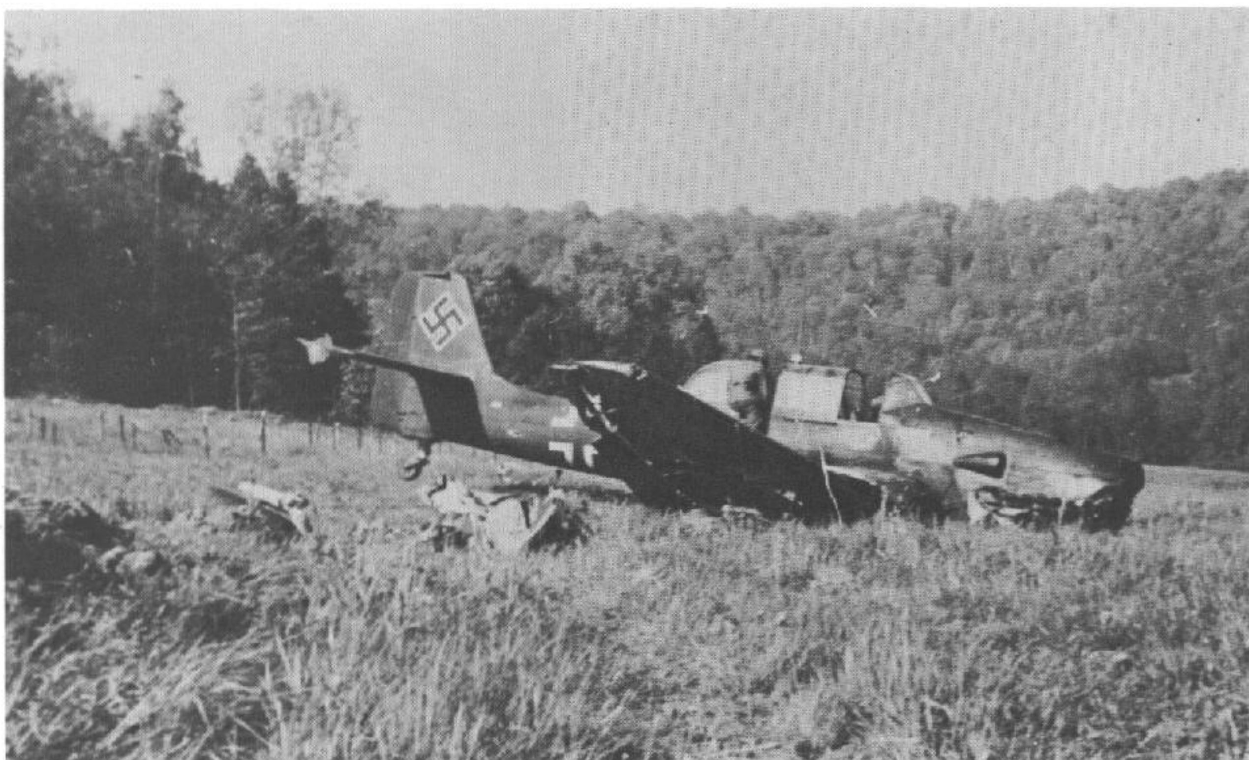
Badly damaged Ju 87 B-1 crashlanded after attacking retreating French Forces in Western France. Part of the nose and the undercarriage are scattered over the field, note holes in rear Fuselage, probably from small arms fire.
